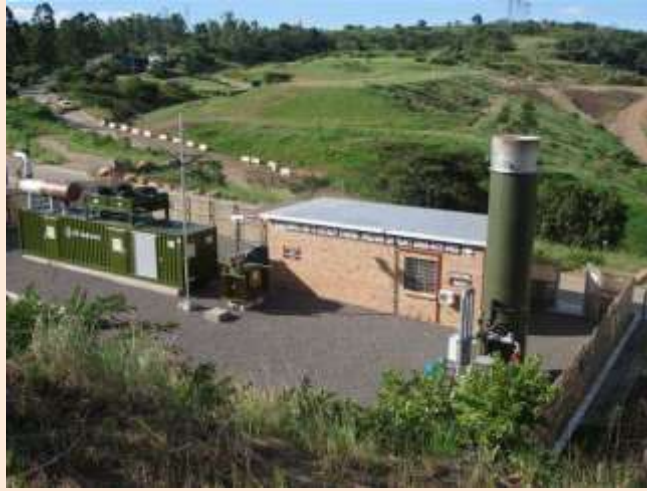
Landfill gas flare at Bisasar Road Landfill Site Mariannahill 1MW LFG to electricity project
