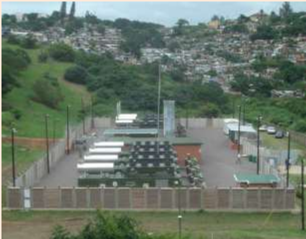
Bisasar Road 6.5MW LFG to electricity project
