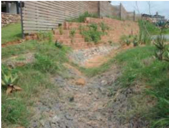
Figure 12: Bio-swale harvesting and stormwater filtration (KZN)
